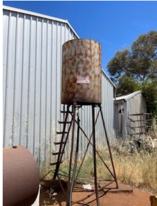
Figure 4: Overhead fuel tank and ground staining next to the large shed at 133 Pitman Avenue
