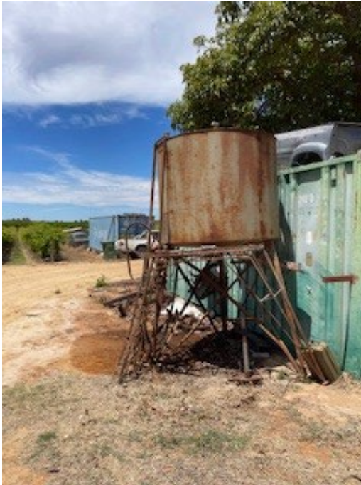
Figure 5: Overhead fuel tank at 90 Melaleuca Street
